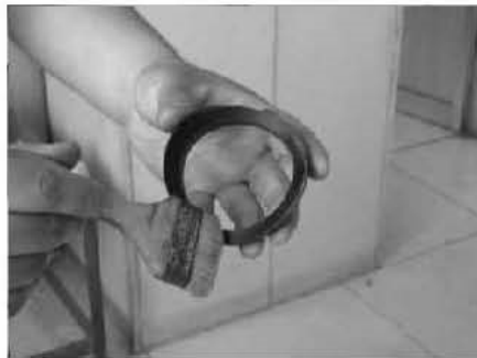
2. Spread lubricant on gasket ring.
