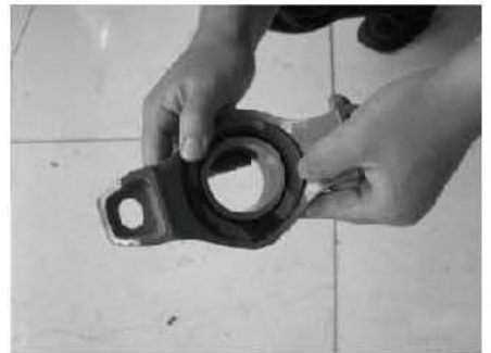
3. Put gasket seal in the Mechanical Tee.
