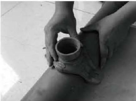
4. Install the Mechanical Tee in the hole.
